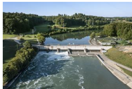
Bannwil Capacity: 28.5 MW End of the concession: 2050
