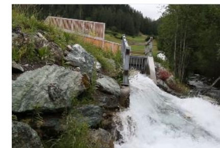
Kraftwerke Ragn d'Err AG Capacity: 7.4 MW End of the concession: 2076
