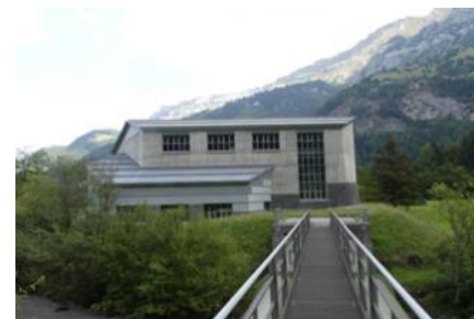
Kandergrund Capacity: 18.8 MW End of the concession: 2071
