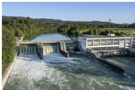
Aarberg Capacity: 15.2 MW End of the concession: 2048
