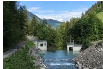
Kraftwerk Spiggebach AG Capacity: 2.9 MW End of the concession: 2097
