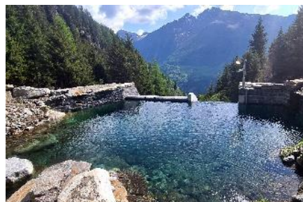
Idro Arvigo SA Capacity: 1.7 MW End of the concession: 2083
