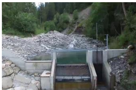
Kraftwerk Fermelbach AG Capacity : 2.0 MW End of the concession: 2096
