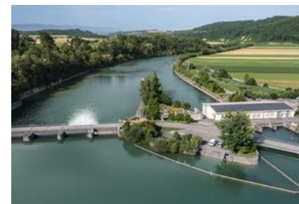
Niederried-Radelfingen Capacity: 15.0 MW End of the concession: 2043
