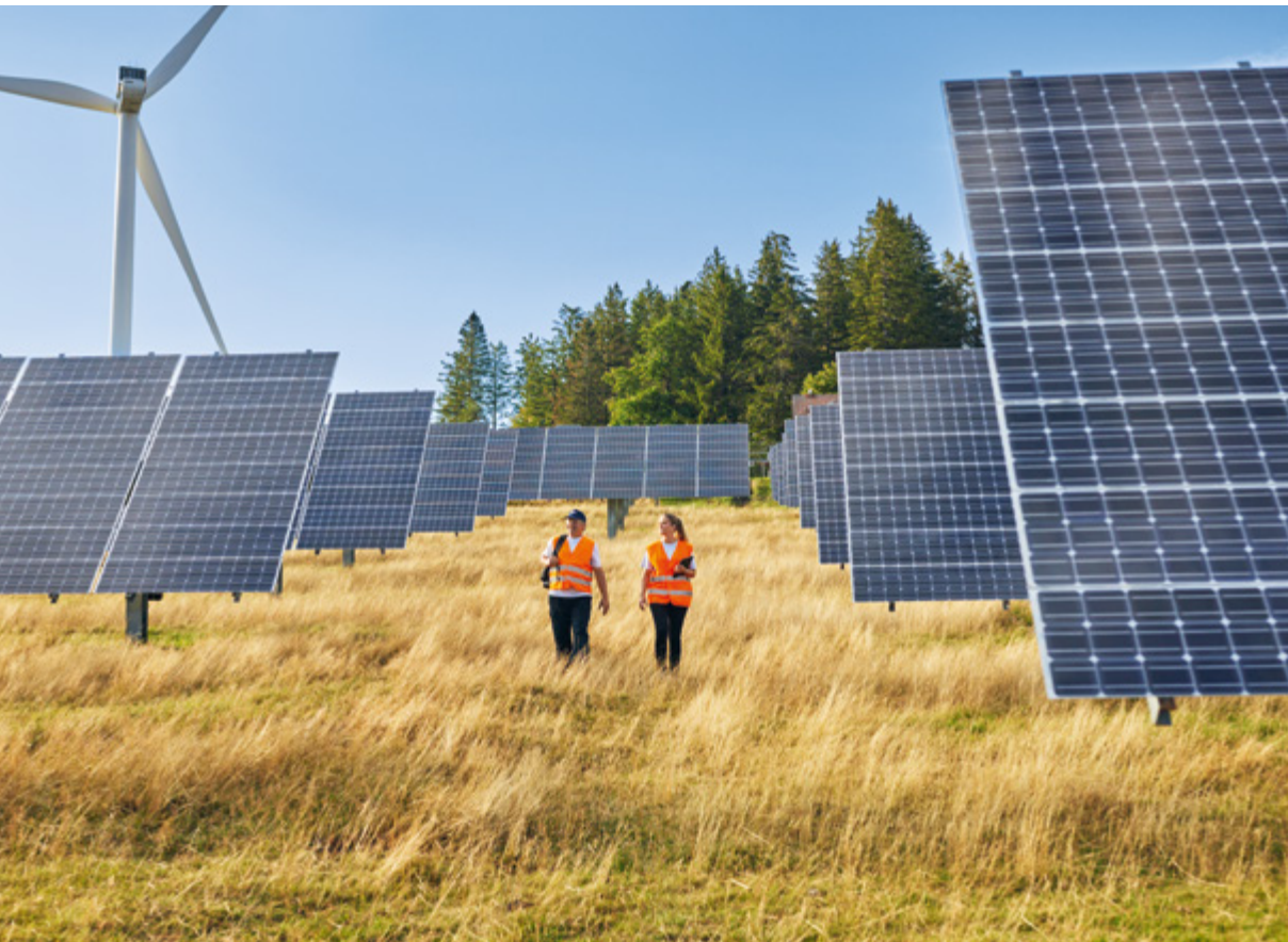
BKW employees check the PV system of the Mont-Soleil solar power plant.
